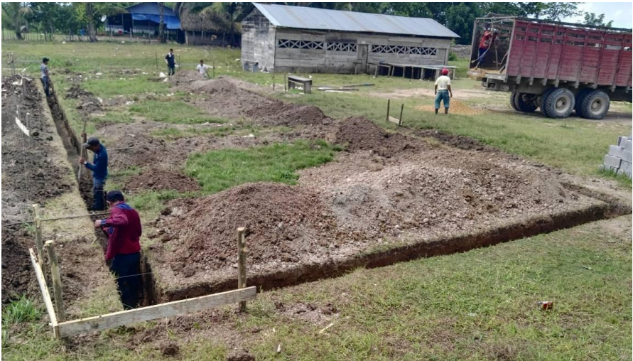
Construction in School of Argentina Community
