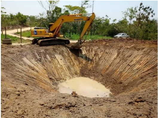
Phase I of reservoir construction.
