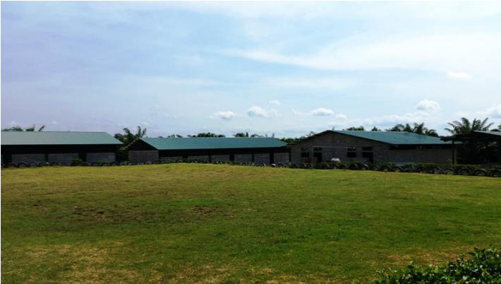
New worker housing buildings and shower facility at the "Union B" housing site.
