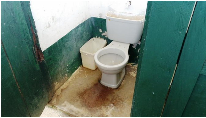
New toilets installed in worker housing.
