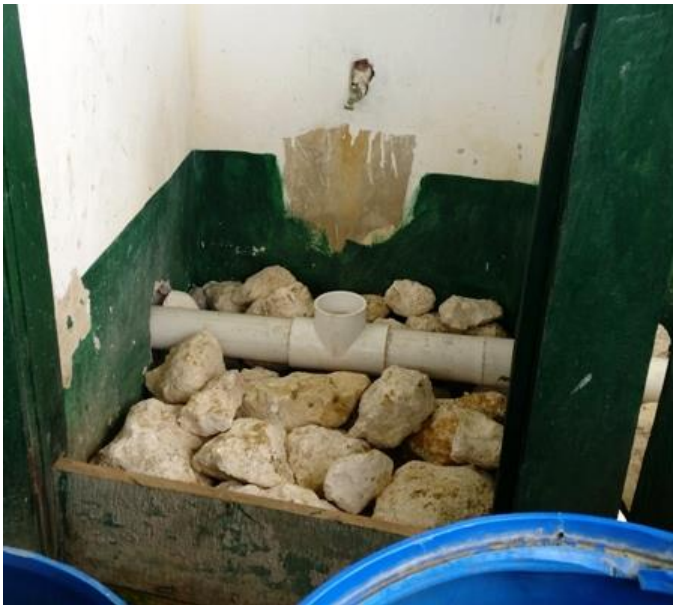
Refurbishing new toilets and connection to wastewater treatment.
