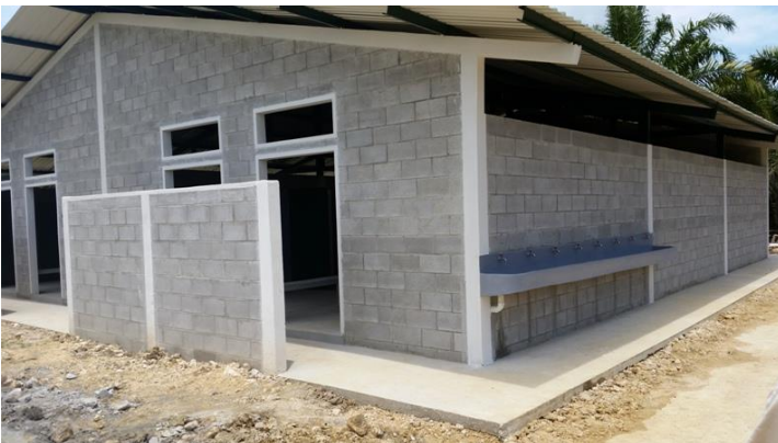
New worker showers and sinks.
