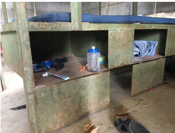
Lockers to be renovated in old dormitories.
