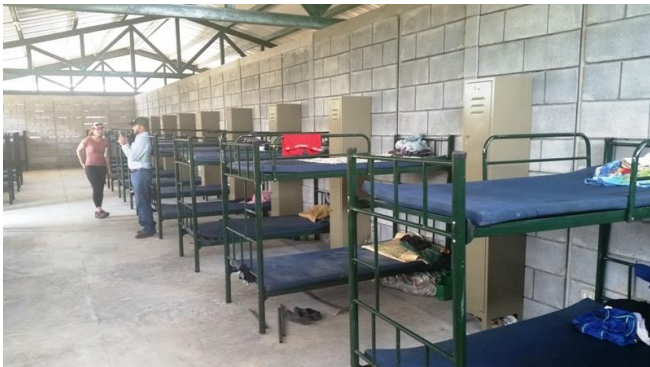
New worker housing building, two-level bunkbeds with safety railing, and lockers.
