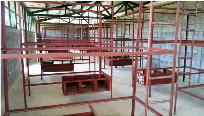
Existing bunkbeds being installed and refurbished in new housing building.
